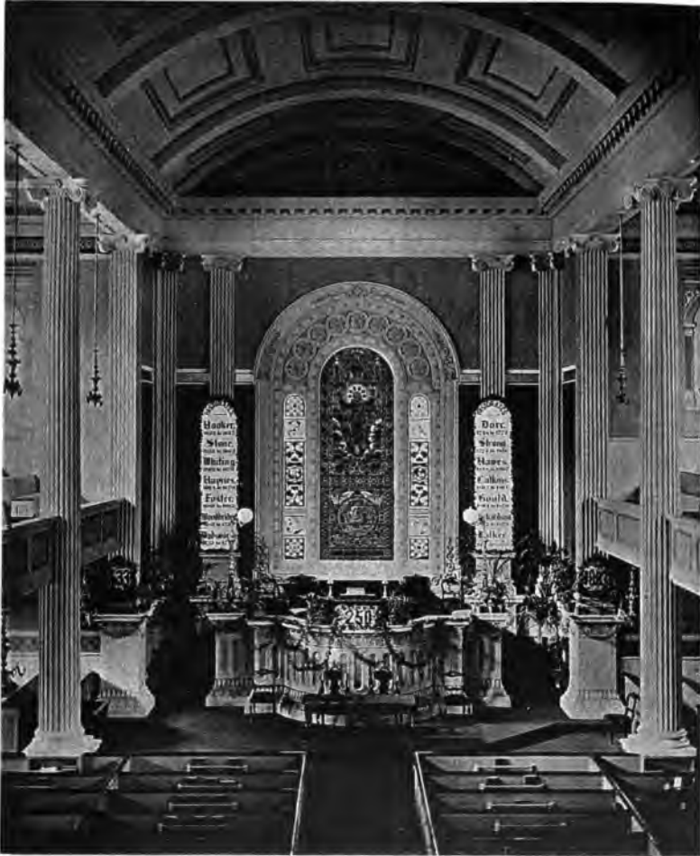
INTERIOR OF FIRST CHURCH.
